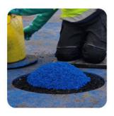
Overfill the area with material to allow for compaction when completing the repair
