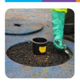
Use the paint brush to apply some of the resin to the edges of the repair, to aid with the bonding of the new material
