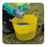
Mix the rubber granules and resin binder in the wheelbarrow / mixing tub to the suggested ratio (refer to page 1)
