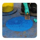
Lubricate the Steel Float with Soapy Water and use to level and compact the material into the repair
