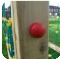
Fastenings are tamper-proof or capped with secure custom-made plastic tamper proof covers. All footholds have a slip-resistant surface.
